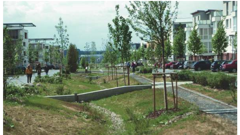
Figure 5. Bioswale in residential POS as an element for stormwater management in Kronsberg settlement
