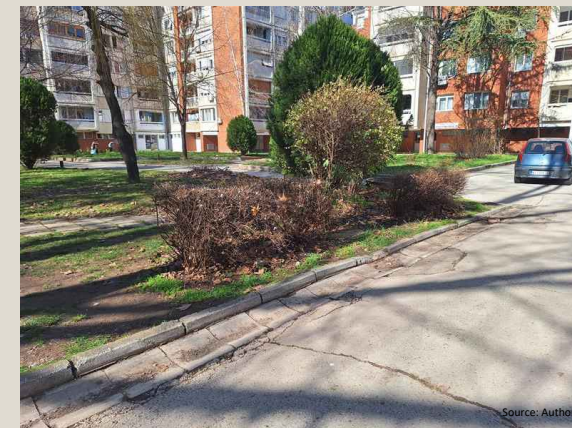
EXISTING CONDITION - BEFORE INTERVENTIONS
