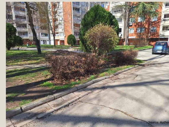
EXISTING CONDITION - BEFORE INTERVENTIONS
